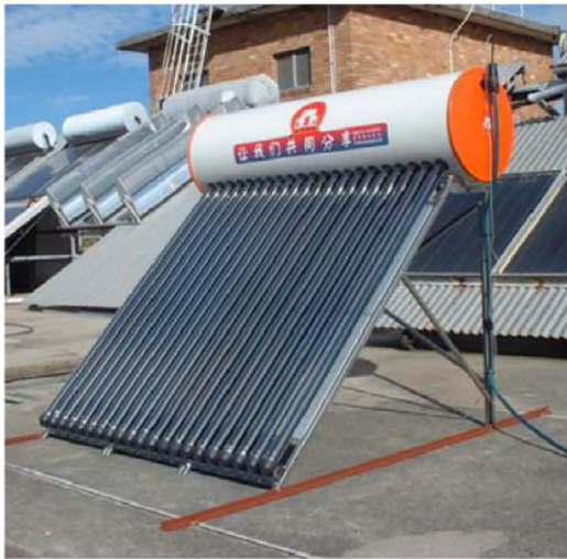
Fig. 5. Schematic and photo of water-in-glass evacuated tube solar water heater [43].
