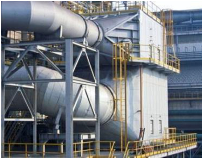
Fig. 3. A functioning heat pipe heat exchanger unit.
