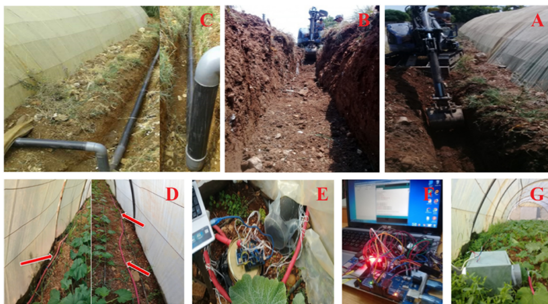
Fig. 4. Stages of conducting the experiment: (A) Excavate the first side, (B) Excavate the second side, (C) Pipes installation, (D) Connecting the wires to the sensors to the tubes, (E) and to the Arduino devices, (F) Connecting with a laptop, and (G) Installation of air intake devices.
