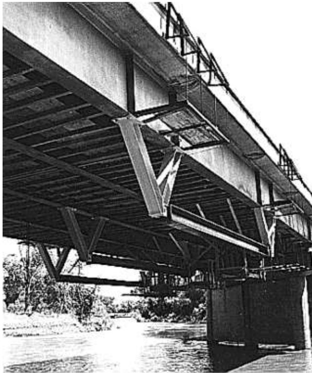
Fig. 22. Highway I-35 Bridge with semi-active dampers [35].
